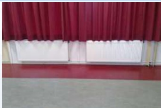
9 | Pakking in radiatoren
